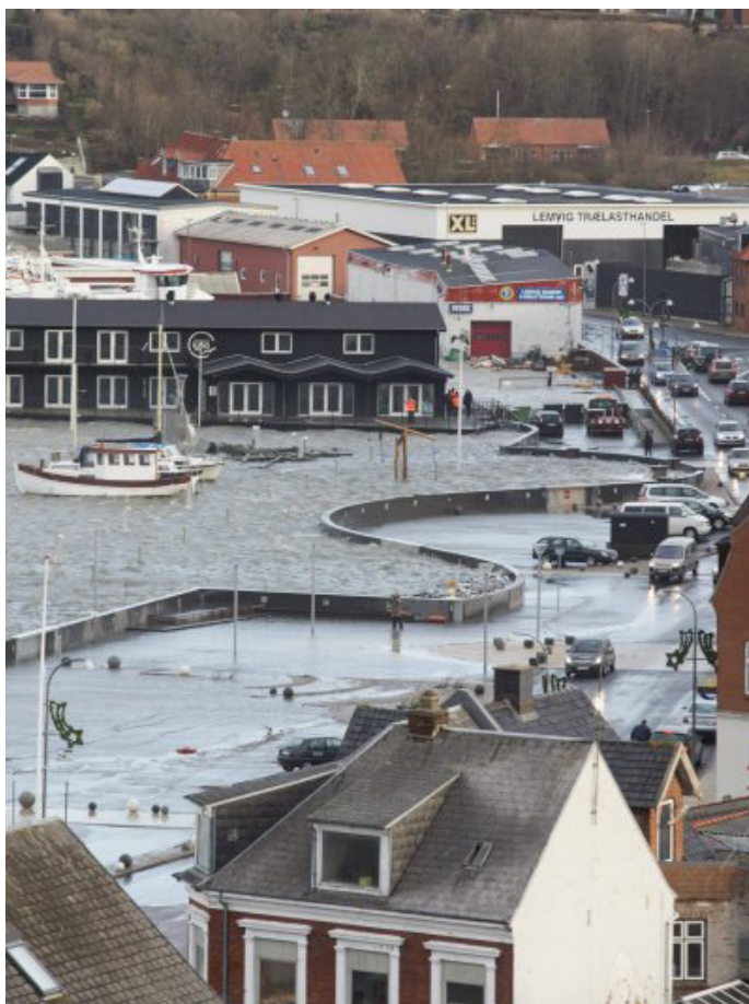
“Le Mur” i Lemvig under stormflod.
